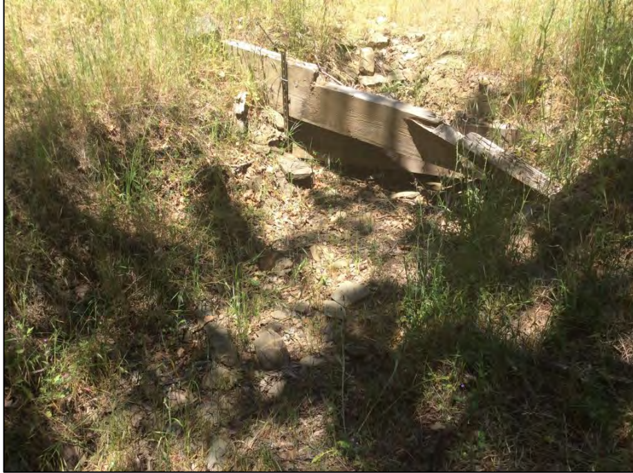
Photo 7. The road crossing over an intermittent section of Upper Penitencia Creek at SC6 that was dry at the time of the May and June field surveys. A small wooden retaining wall stabilizes the downstream side of the road.
