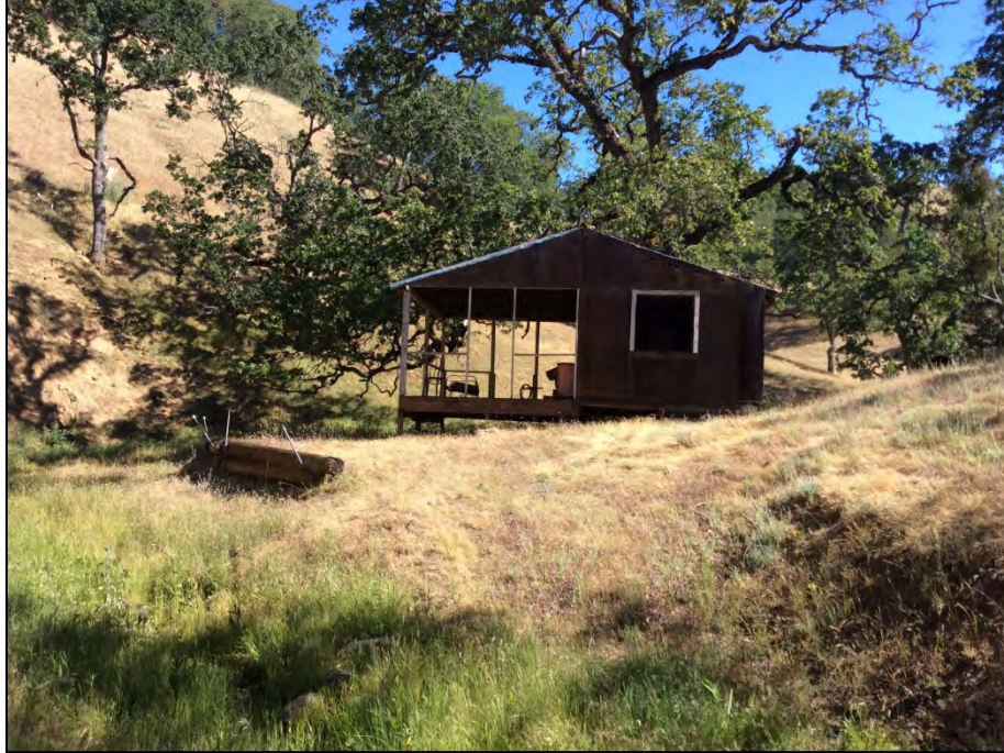
Photo 17. Old one-room ranch house and adjacent retaining wall.
