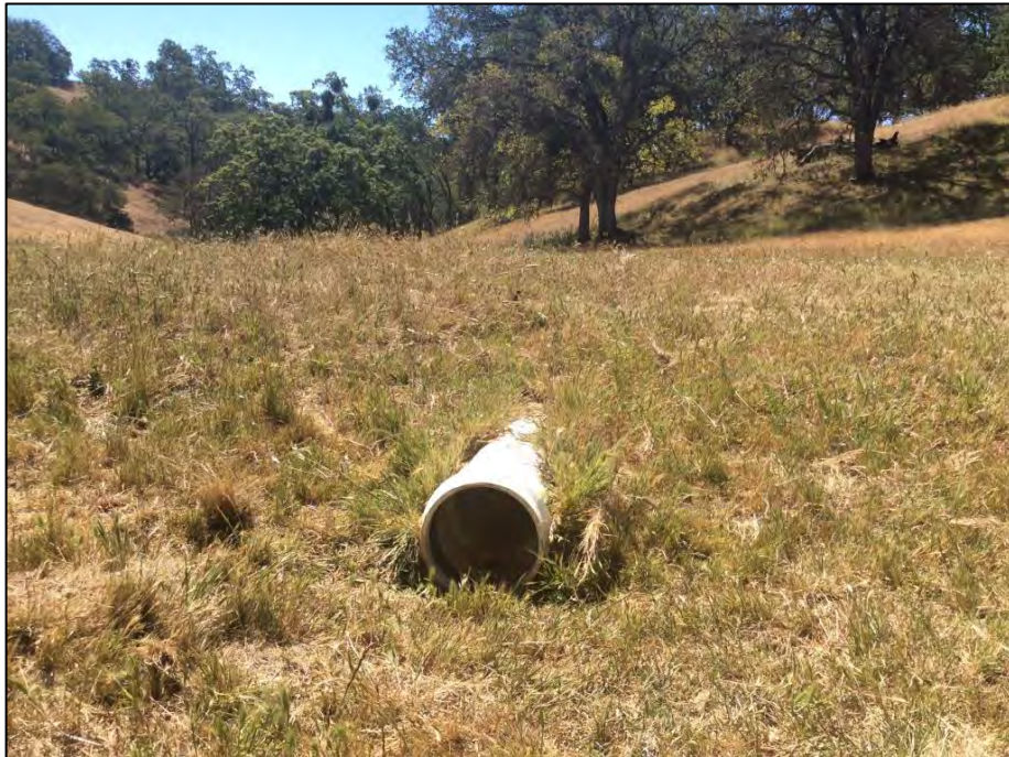
Photo 8. Culvert outlet at SC9.
