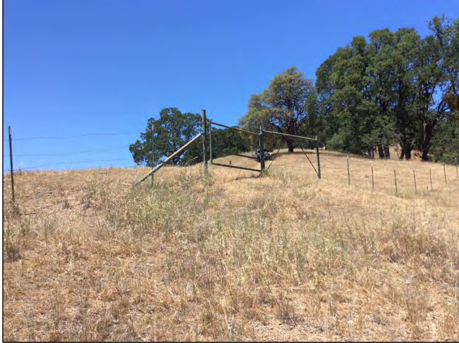
Photo 11. Barbed wire fence and gate to exclude cattle from Pond 4.
