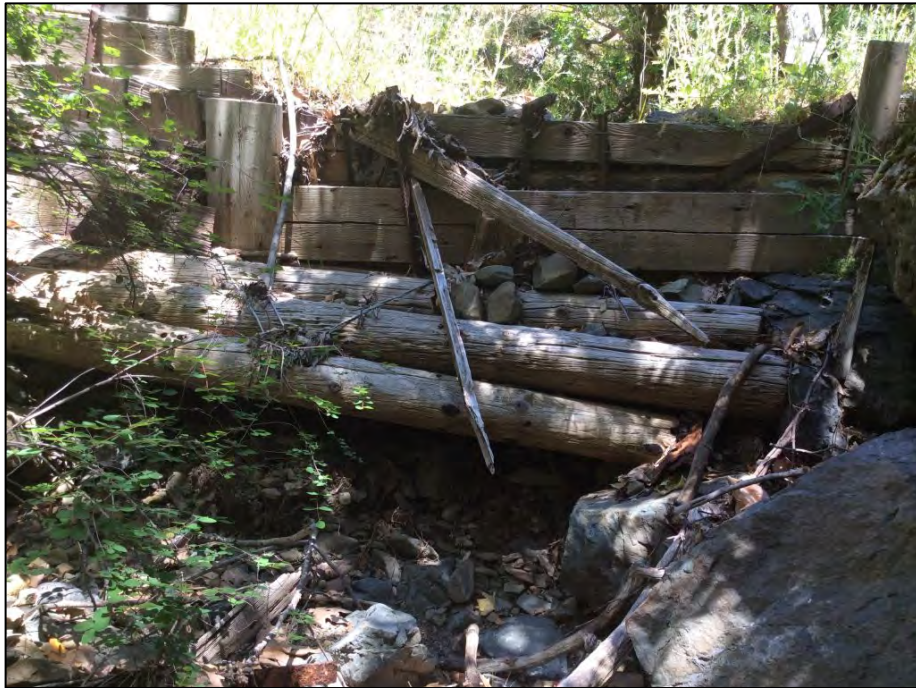
Photo 6. A wooden retaining wall stabilizing the downstream side of SC3.
