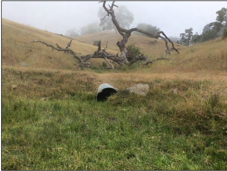
Photo 9. Culvert outlet at SC10.
