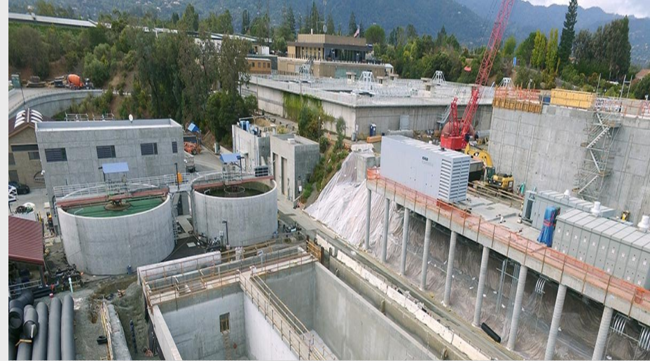
RWTP Reliability Improvements ($290 Million)
