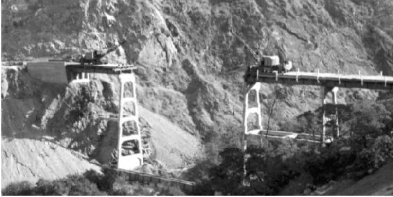
Construction at Anderson Reservoir, 1951
