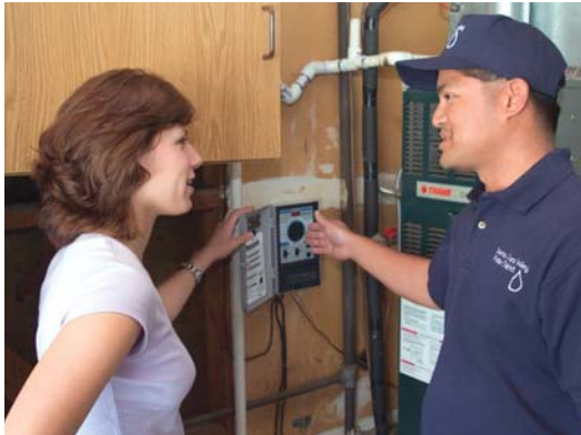
A Water-Wise House Call technician looks at an irrigation controller with a resident.
