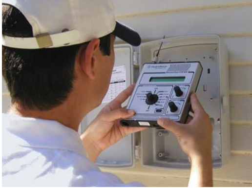
Water conservation technician programs evapotranspiration (ET) irrigation controller.
