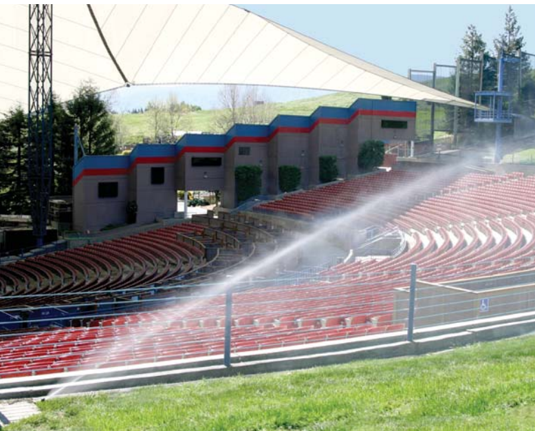
Irrigation system evaluation at Shoreline Amphitheater.
