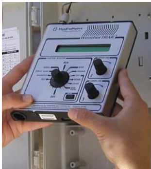
Installation of evapotranspiration (ET) irrigation controller.
