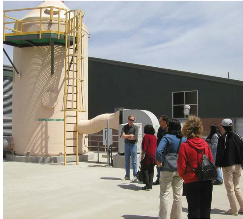
Educational tour to Alameda County Water District's brackish desalination facility.
