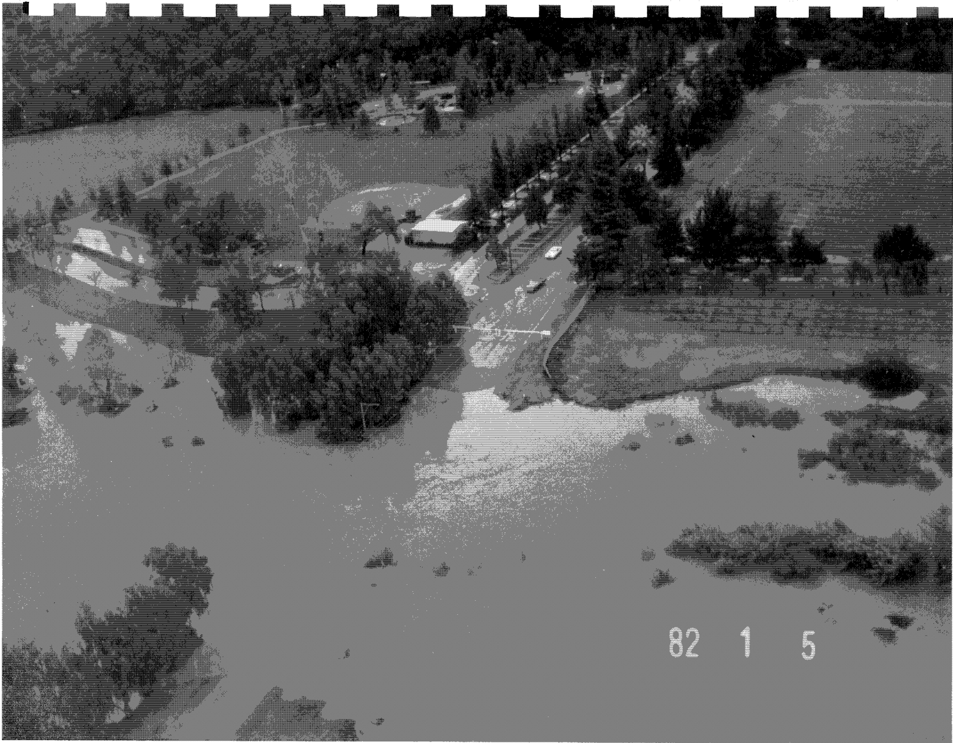
UVAS CREEK FLOODING MILLER AVE. CROSSING 1/5/82
