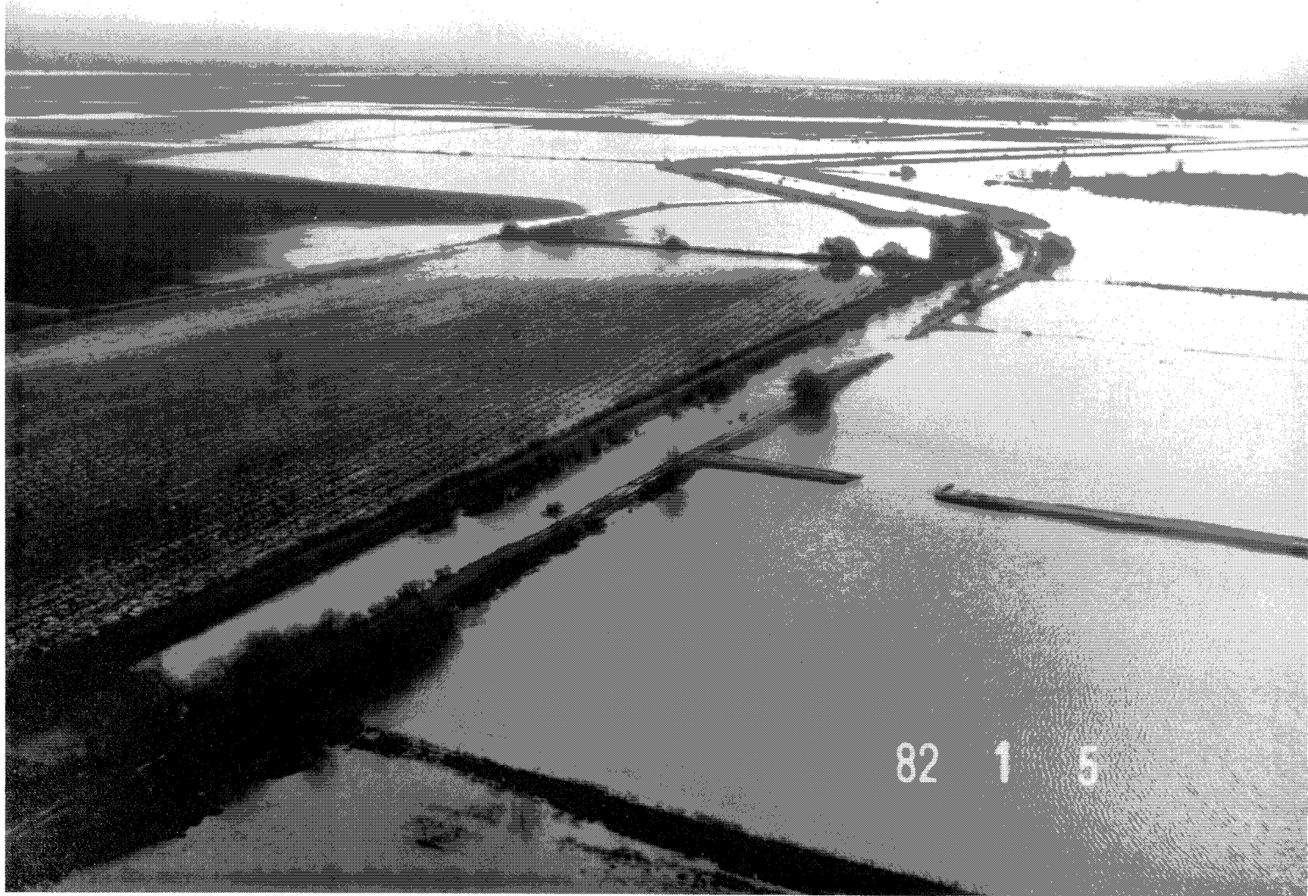
LLAGAS CREEK FLOODING GILROY SEWAGE FARM LEVEE BREAK NORTH OF BLOOMFIELD RD.
