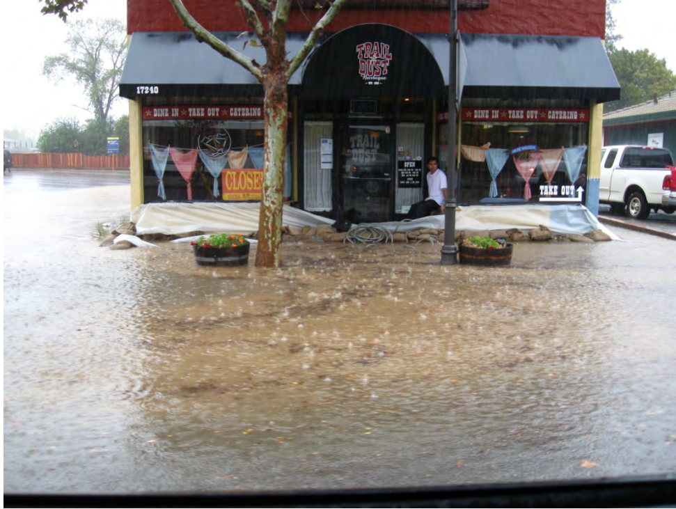
Photo 7: Flooding around Trail Dust Restaurant in Morgan Hill. Photo courtesy Anthony Eulo, Program Administrator, Environmental Services Department of the City of Morgan Hill.
