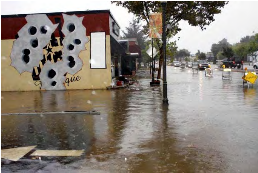
Photo 8: The parking lot just north of Trail Dust floods as a result of the Oct. 13 storm. Photo by Jorge Briones
