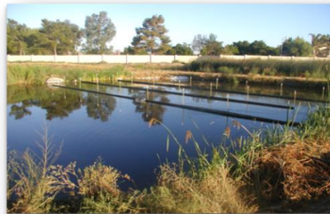
Treatment by Engineered Wetland
