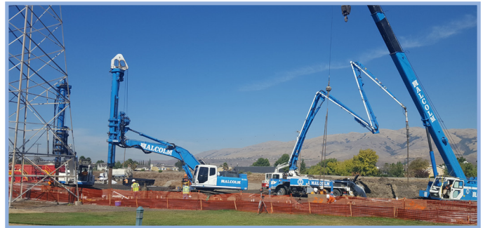
Example of the pile foundation work.
