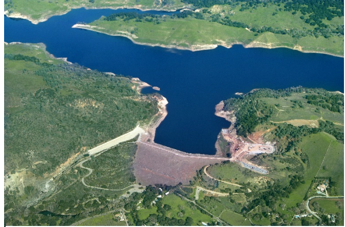
Anderson Reservoir is currently being operated at 52% of capacity due to seismic concerns with the dam at full capacity.
