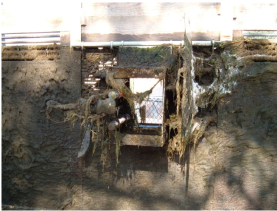
Figure 3. Alamitos Fishway deployment 2003-2004 Note small flow through weirs on sides.
