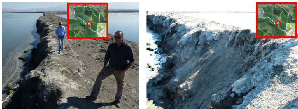
Figure 9 - Steepen dry silts and resulting sliding
