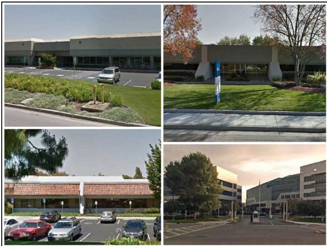
Figure 10. Representative Commercial and Industrial Structures in EIAs 7, 8, and 9
