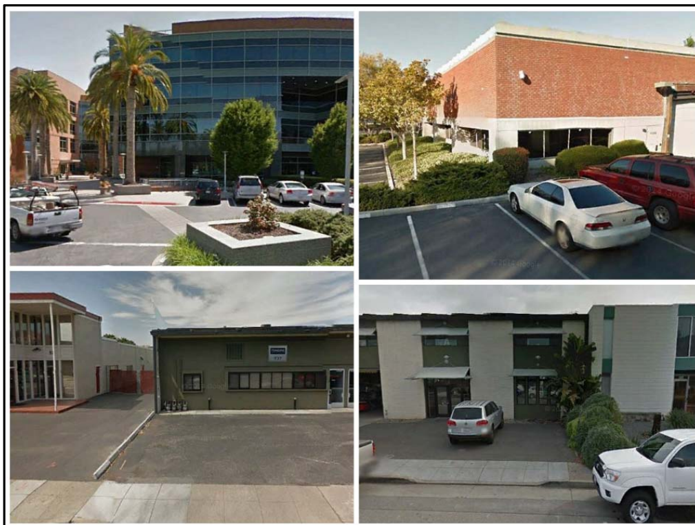
Figure 9. Representative Commercial and Industrial Structures in EIAs 4 and 5
