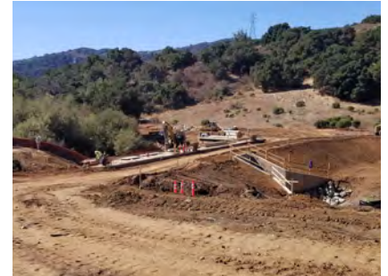
Construction of the Control Structure at Rancho San Antonio
