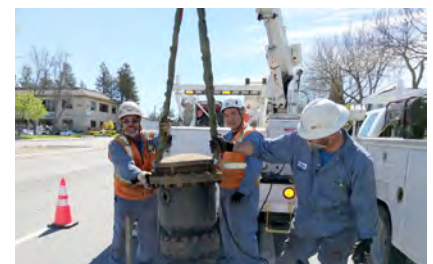
Parallel East Pipeline Refurbishment
