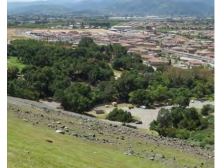
Anderson Dam during Division of Safety of Dams (DSOD) inspection
