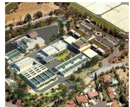
RWTP Reliability Improvement
