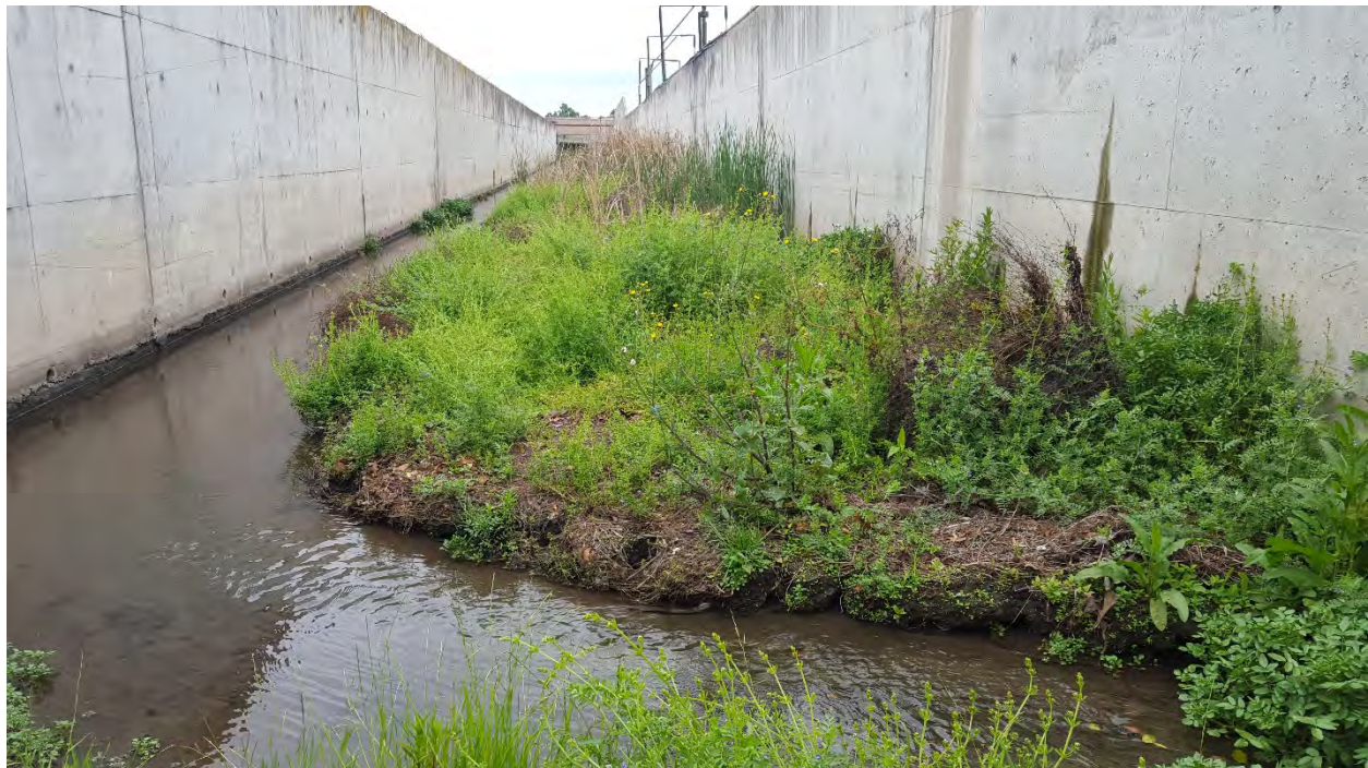
Figure 3: Photographs of Existing U-frame in Reach A
