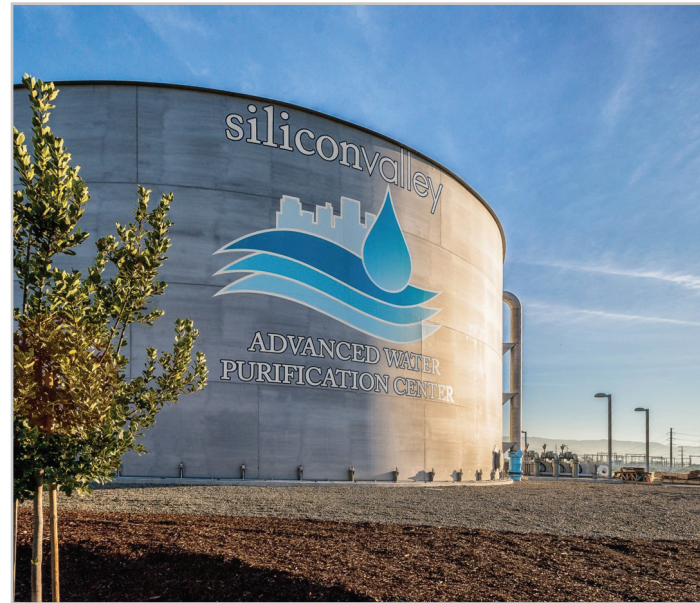
Silicon Valley Advanced Water Purification Plant.
