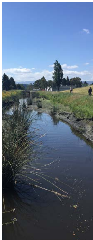
Sunnyvale West Channel from Carl Road looking south to Caribbean Drive
