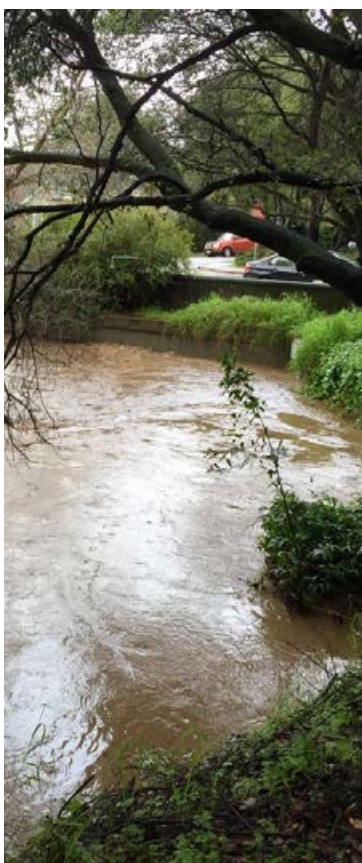
High flows under the Pope/Chaucer Street Bridge
