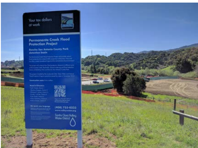
2012 Safe, Clean Water Program - Construction of Rancho San Antonio detention basin, which is part of the Permanente Creek Flood Protection Project.
