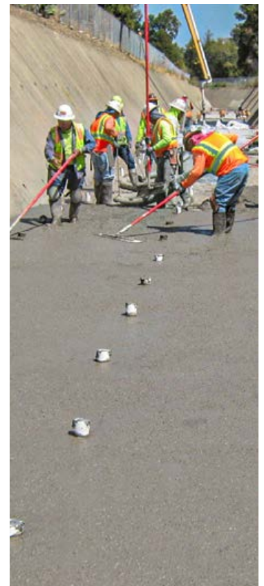
San Tomas erosion repair.
