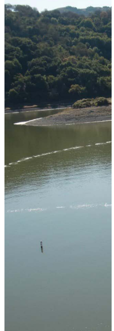
Calero Reservoir Oxygenation System
