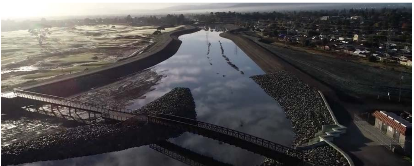
2012 Safe, Clean Water Program: Looking upstream from the Friendship Bridge at the completed portion of the San Francisquito Creek Flood Protection Project from S.F. Bay to Highway 101
