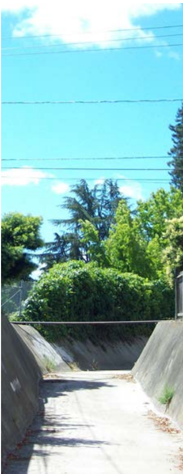
Hale Creek will be the pilot project to restore natural functions and stream stability.
