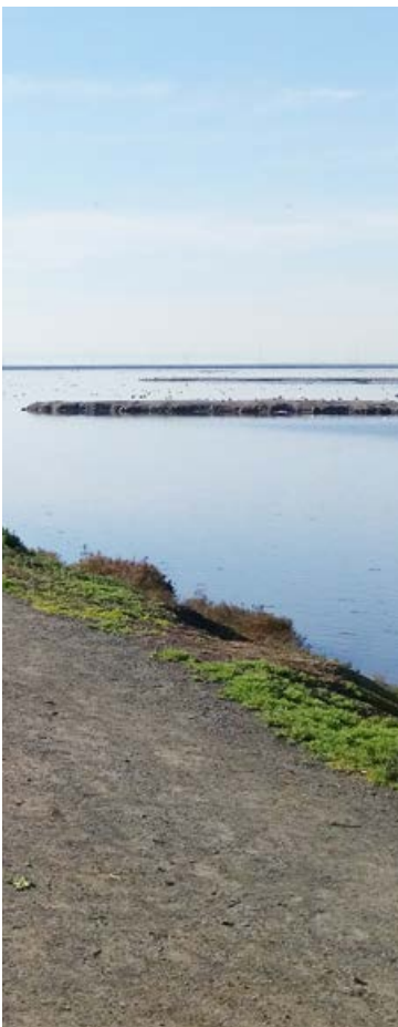
Shoreline Phase 1 levee
