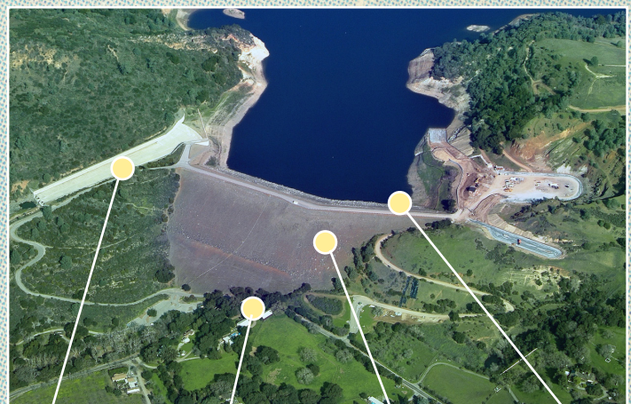
Spillway Outlet pipe Dam embankment Crest of dam
