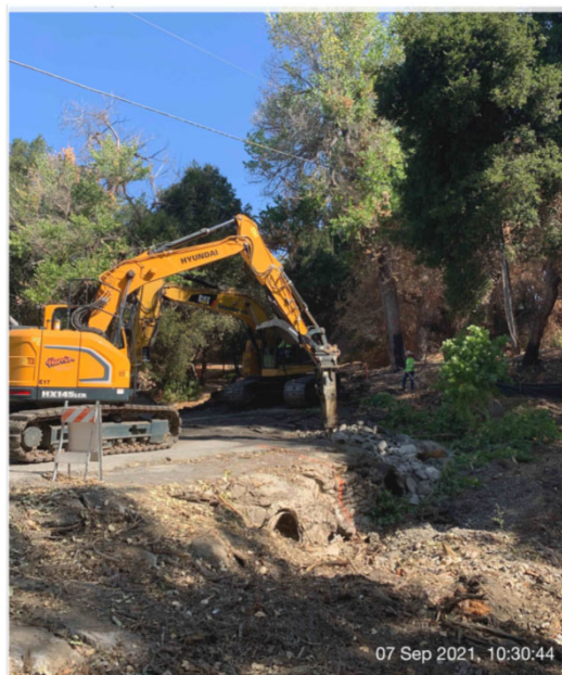
Demolition of the existing crossing
