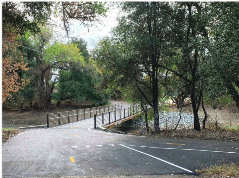
Completed Interim Project
