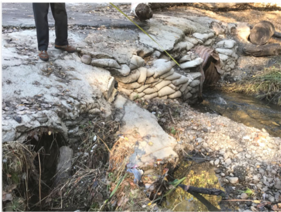
Culvert inlet at upstream face of crossing
