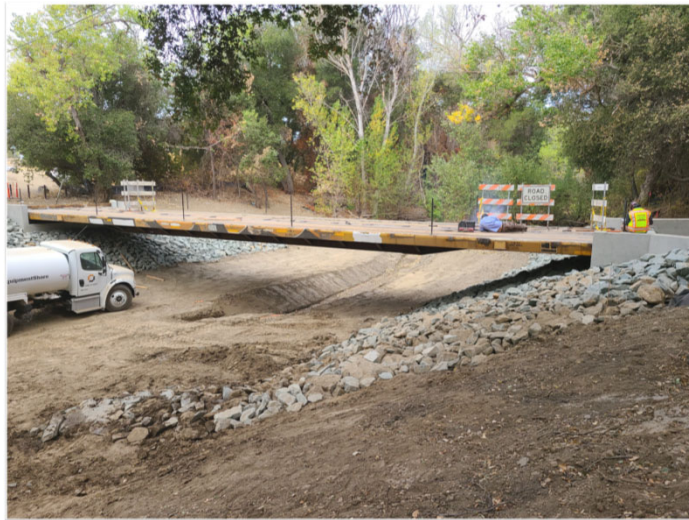
Flow forcing features for fish safety
