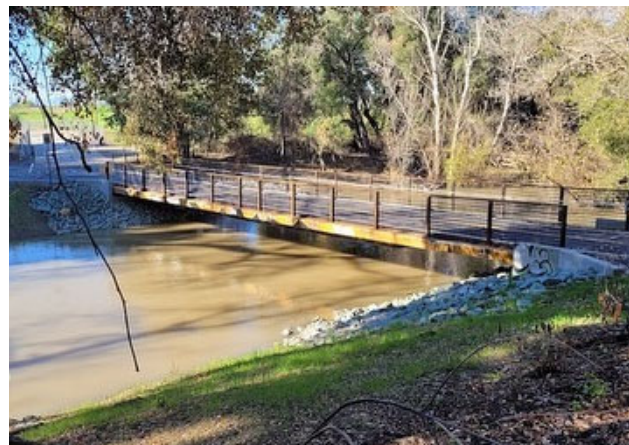
View of new Singleton Road flat car bridge road from upstream with about 300 cfs
