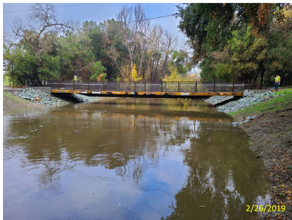
View of new Singleton Road flat car bridge road from upstream with about 300 cfs
