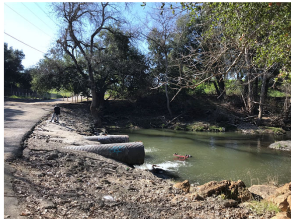
Culvert outlet at downstream face of crossing
