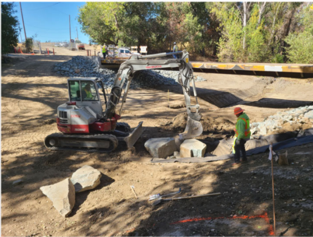
Flow forcing features for fish safety
