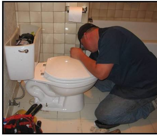
Fixture Replacement Program
