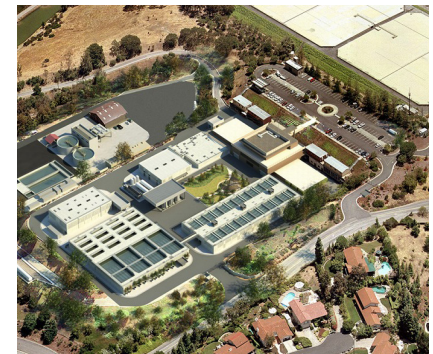
RWTP Reliability Improvement
