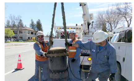
Parallel East Pipeline Refurbishment
