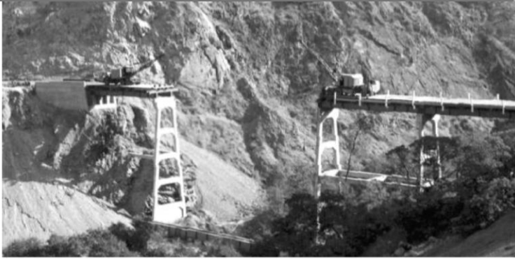
CONSTRUCTION AT ANDERSON RESERVOIR, 1951
