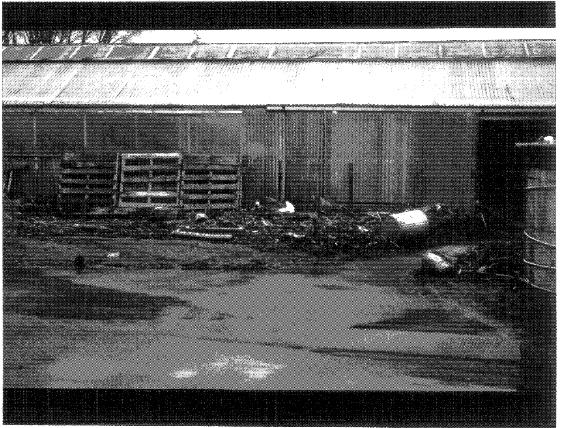
FLOODING DAMAGE CAUSED BY UPPER PENITENCIA CREEK AT KING RD. NURSERY 1/11/95
