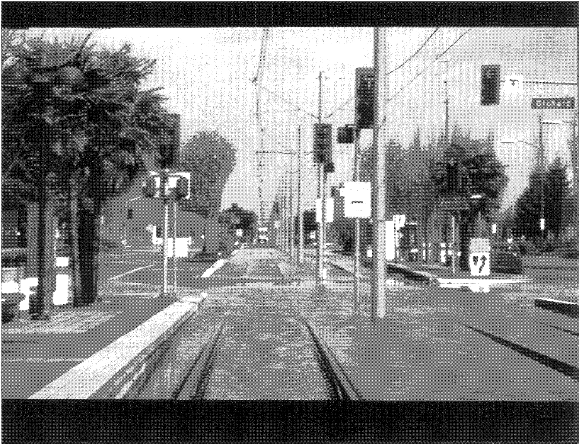
LOCAL DRAINAGE CAUSED BY GUADALUPE RIVER ON THE LIGHT RAIL AT ORCHARD ST. AND FIRST ST. 3/11/95
