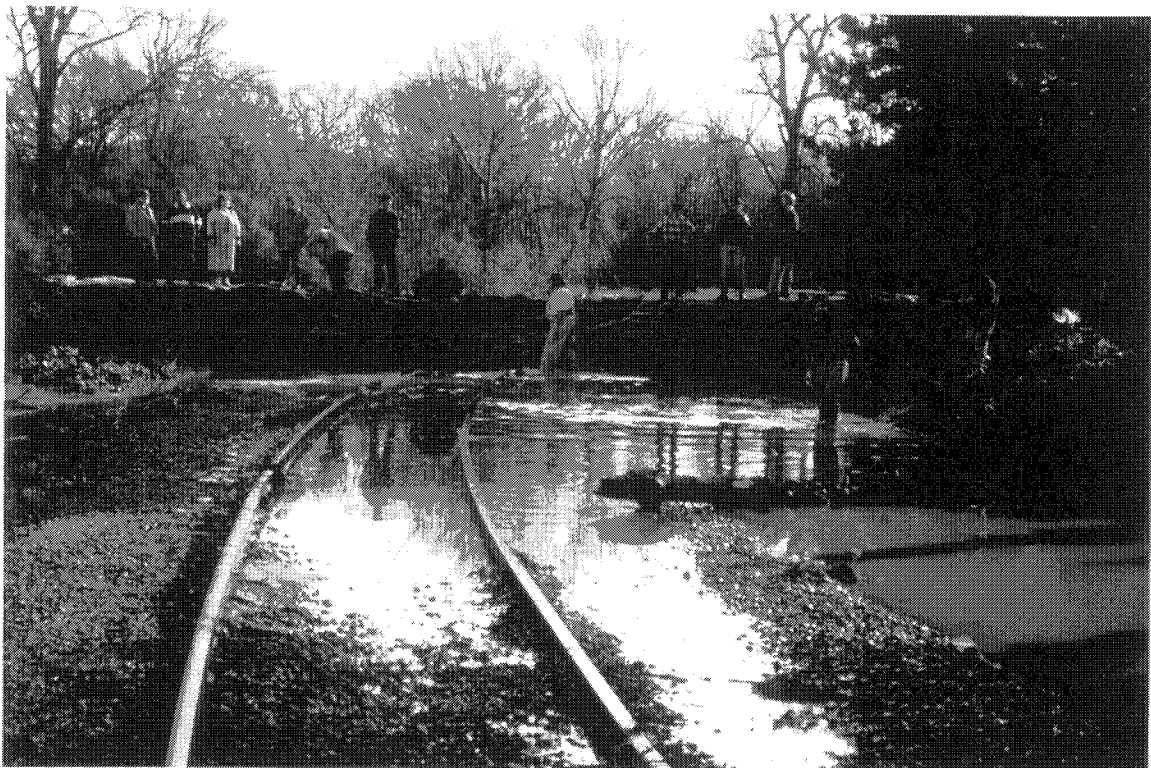
Coyote Creek in San Jose - finished sandbag levee at railroad crossing in San Jose 1-26-97 (S5074-19)
