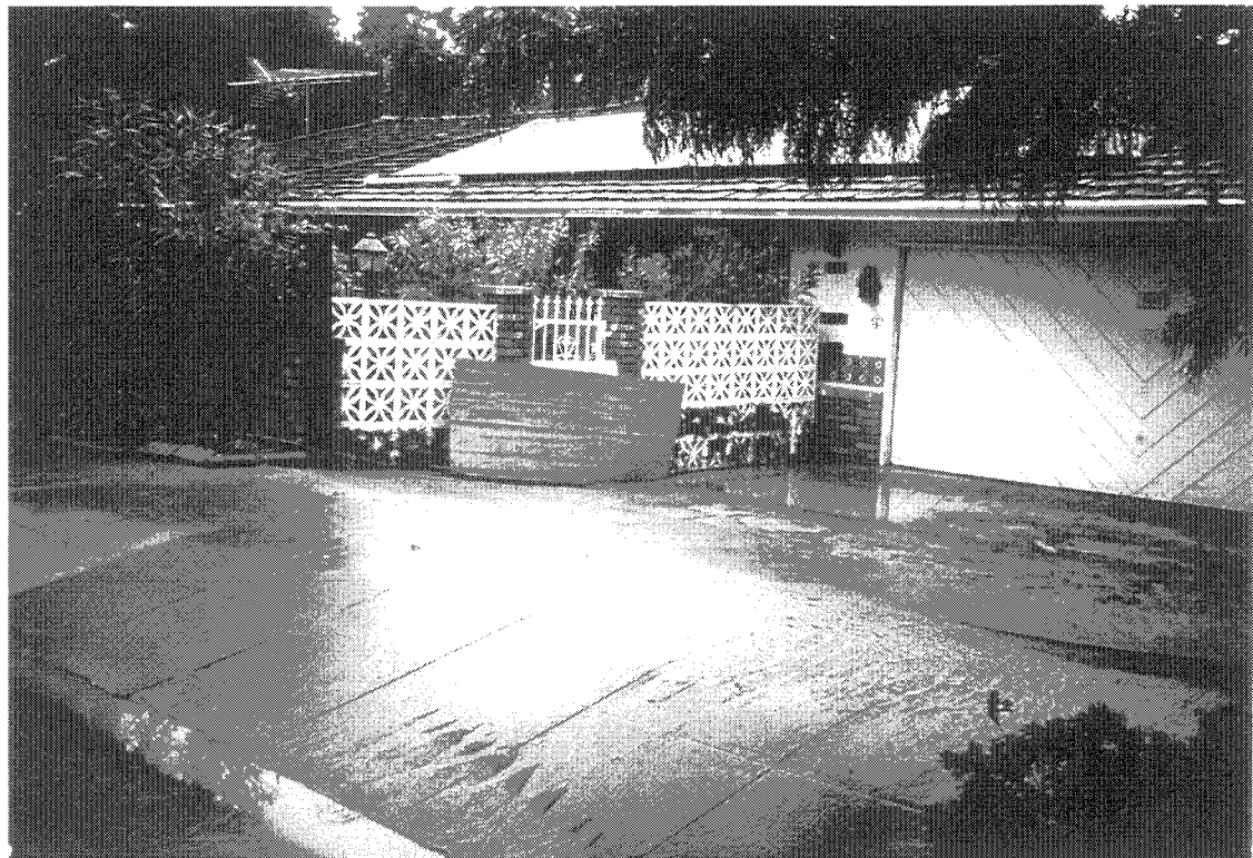
High water mark on fence and mud deposited by San Francisquito Creek flood waters (Palo Alto Avenue in Palo Alto) 2-3-98 (S5199-2)
