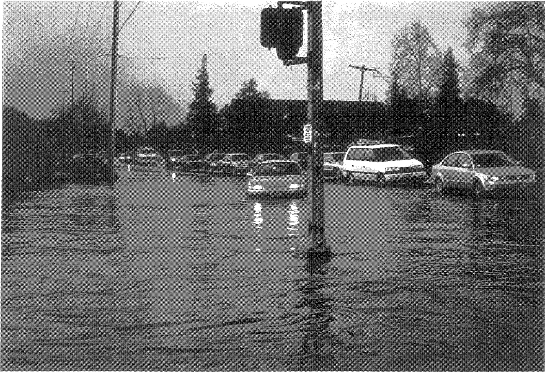
Flooding from Calabazas Creek on Bollinger Avenue in San Jose 2-7-98 (S5184-12)
