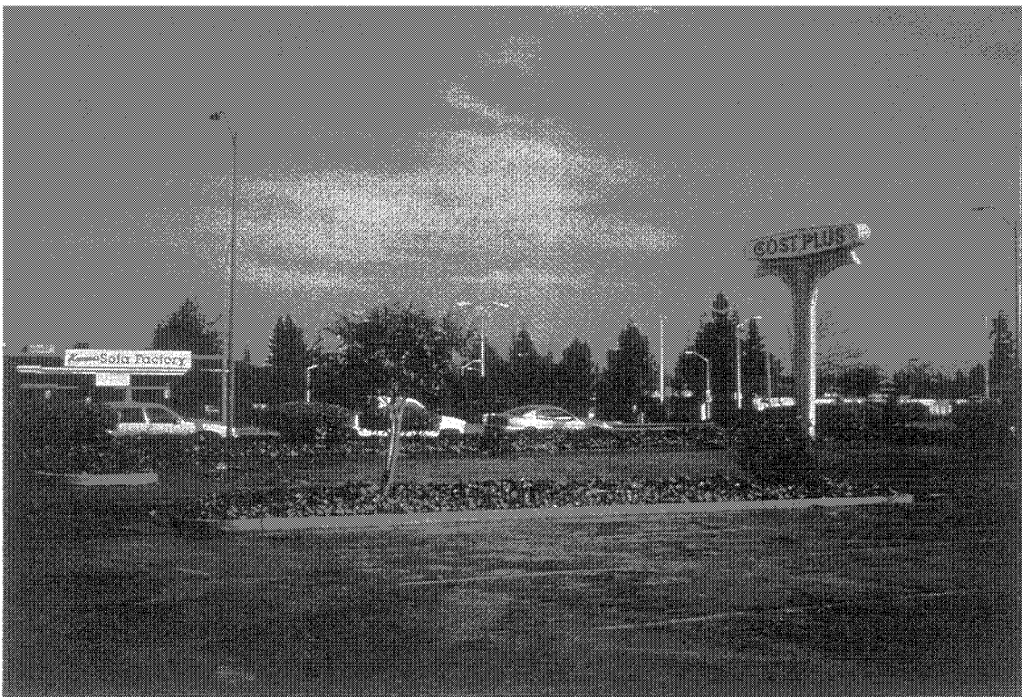
Mud deposited by flood waters from Calabazas Creek in parking lot of business along Stevens Creek Boulevard in Cupertino
