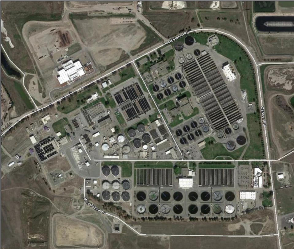
Figure 6: Aerial View of Wastewater Facility
