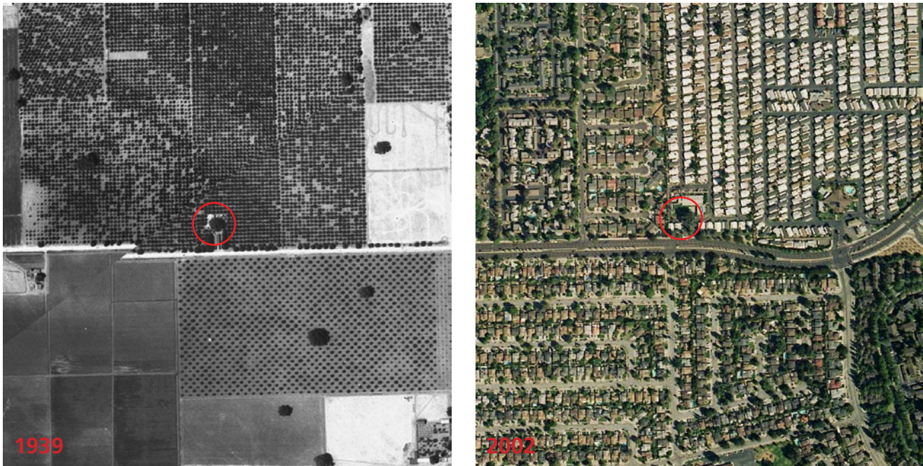
FIGURE II-27. BLOSSOM HILL ROAD IN 1939 (LEFT) AND 2002 (RIGHT). Aerial photographic overlay allows the identification of at least one persisting, heritage oak tree, shown in FIGURE II-28 (AAA 1939; 2002 imagery copyright 2005 AirPhotoUSA, LLC, All Rights Reserved).
