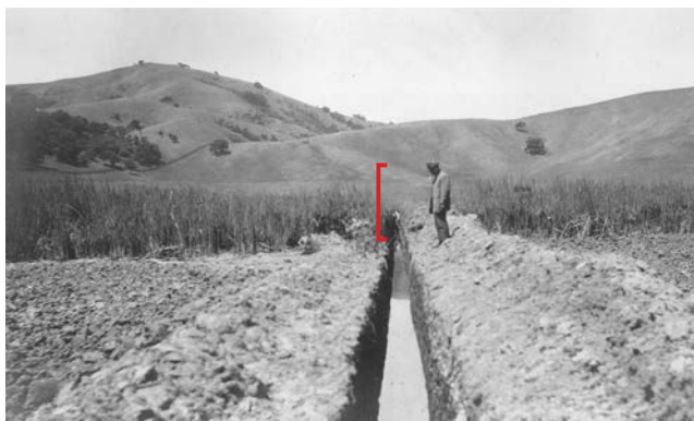
FIGURE II-10. “WATER STOOD FIVE FEET ABOVE GROUND SURFACE BEFORE RECLAMATION” [text from original photo caption]. Photograph taken immediately following the construction of drainage ditches through Laguna Seca (SCVWD Vault 1917).
