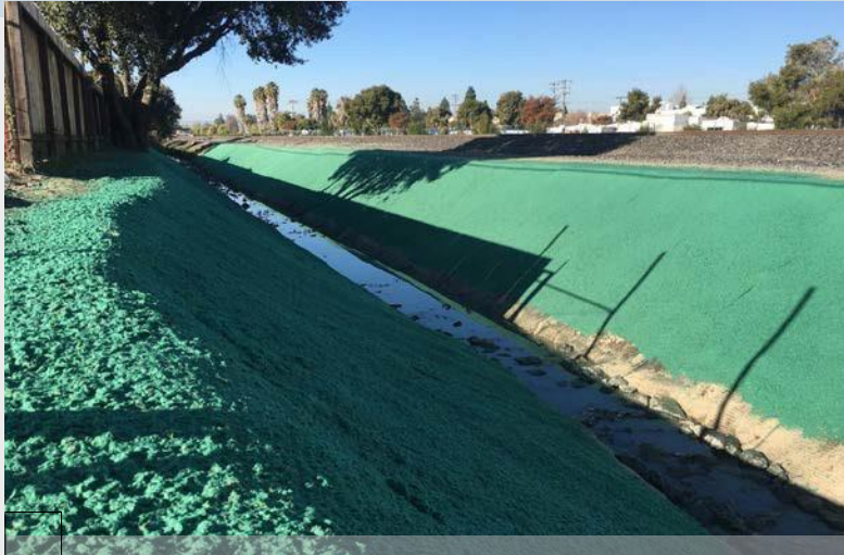
Watershed Asset Rehabilitation Program
