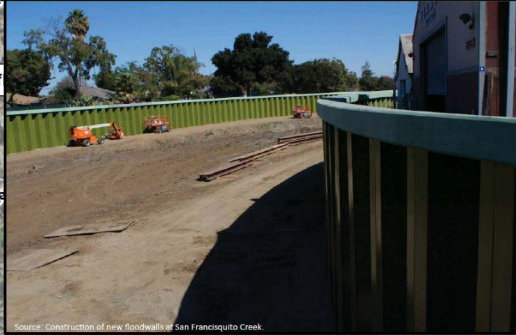
Source: Construction of new floodwalls at San Francisquito Creek
