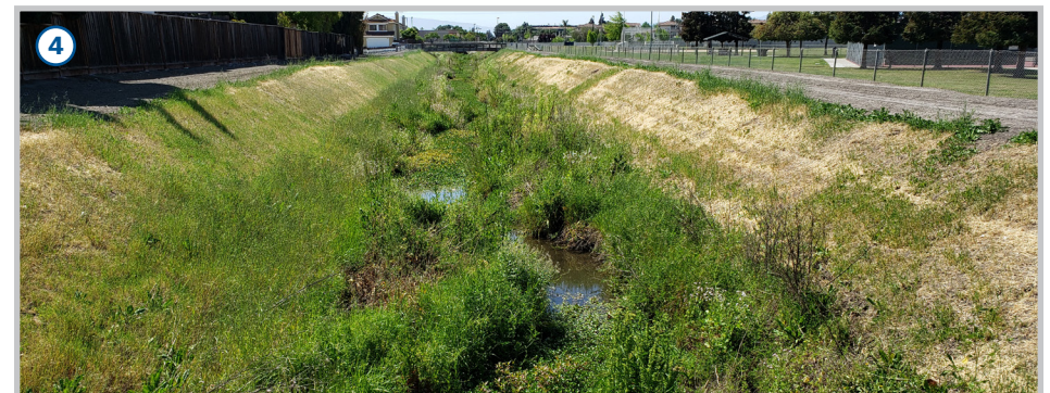
Tularcitos Creek looking downstream from Pacheco Drive.
