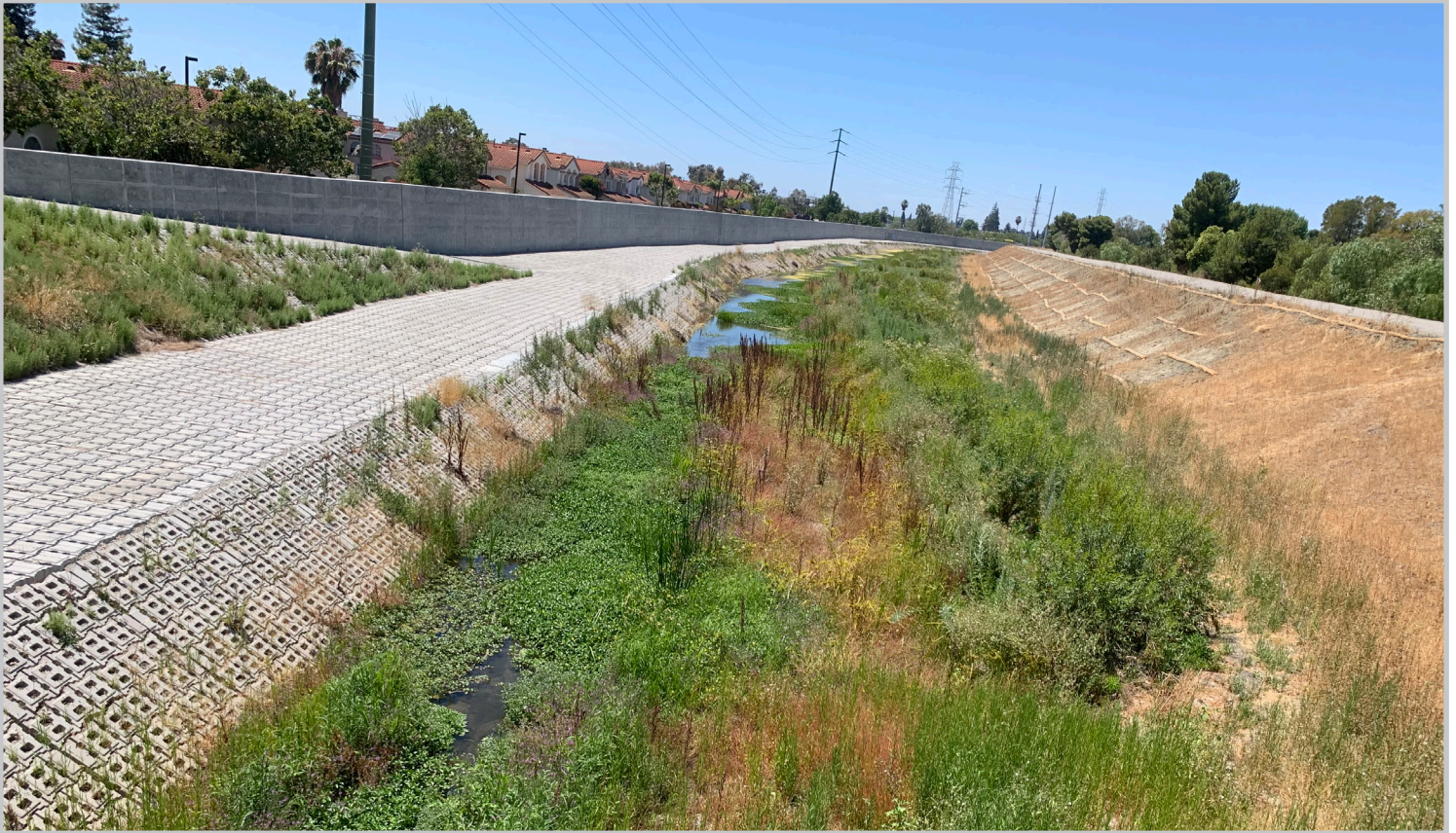
View from N. Milpitas Boulevard looking downstream.
