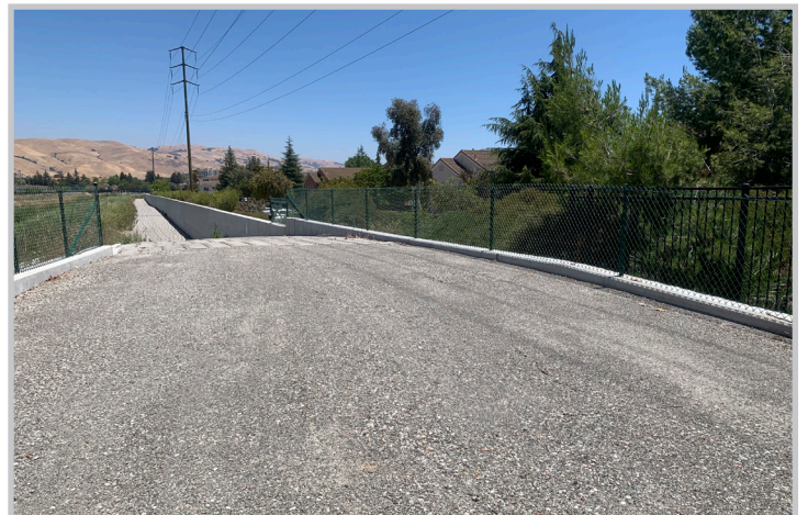
View from N. Milpitas Boulevard looking upstream.
