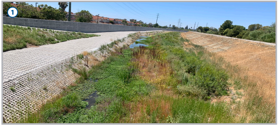
Downstream view of Lower Berryessa Creek from N. Milpitas Boulevard.
