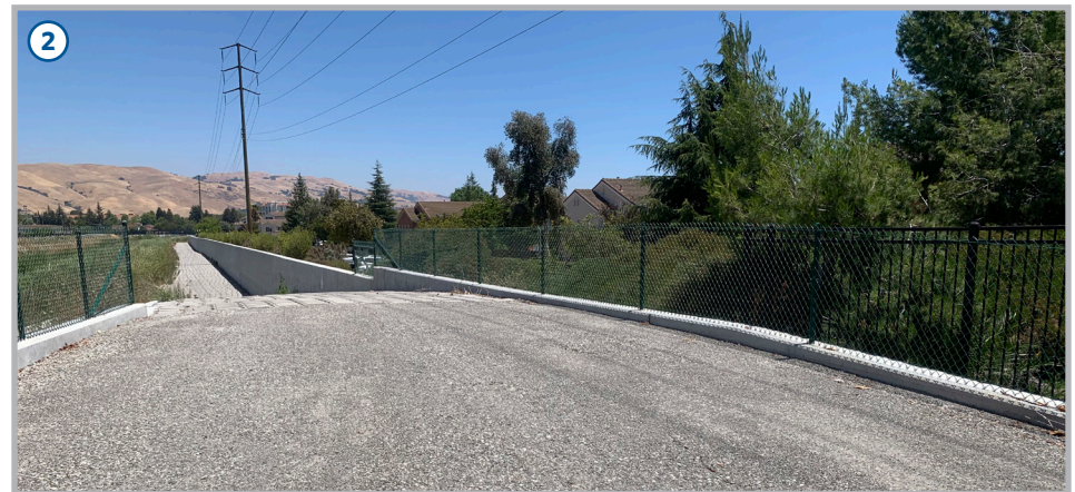
Upstream view of Lower Berryessa Creek from N. Milpitas Boulevard.
