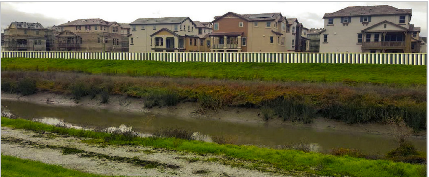
Photo rendering of the steel sheet pile floodwall, the structure located by the Waterstone Development.
