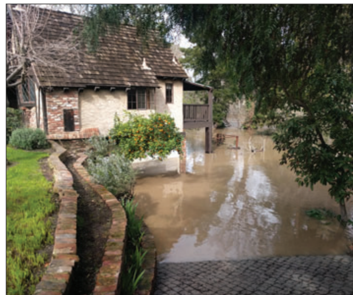
Driveway flooding. Photo: Valley Water
