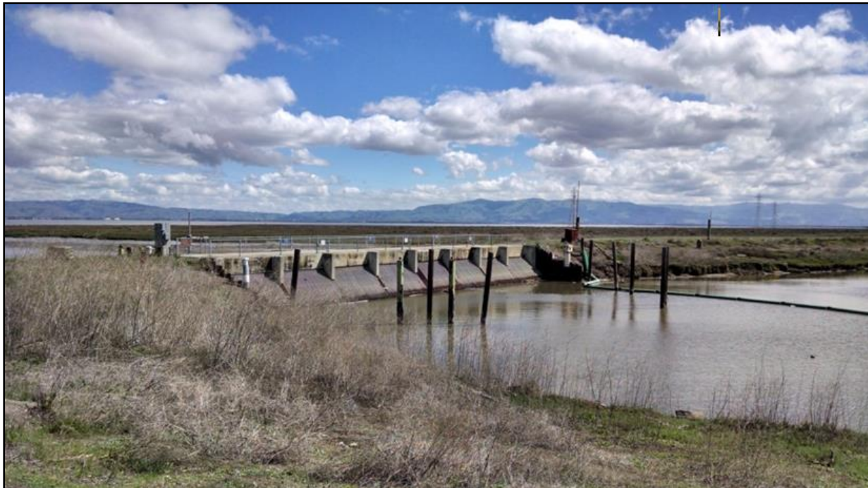
Figure 3-1. Photo of Existing Tide Gate and Levee
