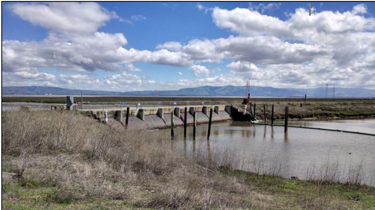
Figure 3-1. Photo of Existing Tide Gate and Levee
