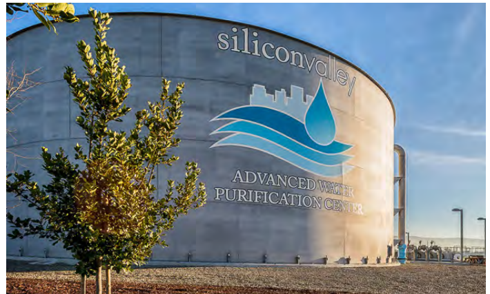
Silicon Valley Advanced Water Purification Center
