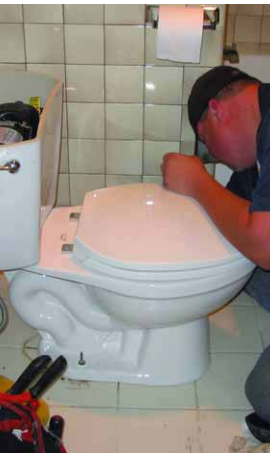
Technician installs High-Efficiency Toilet in restaurant.
