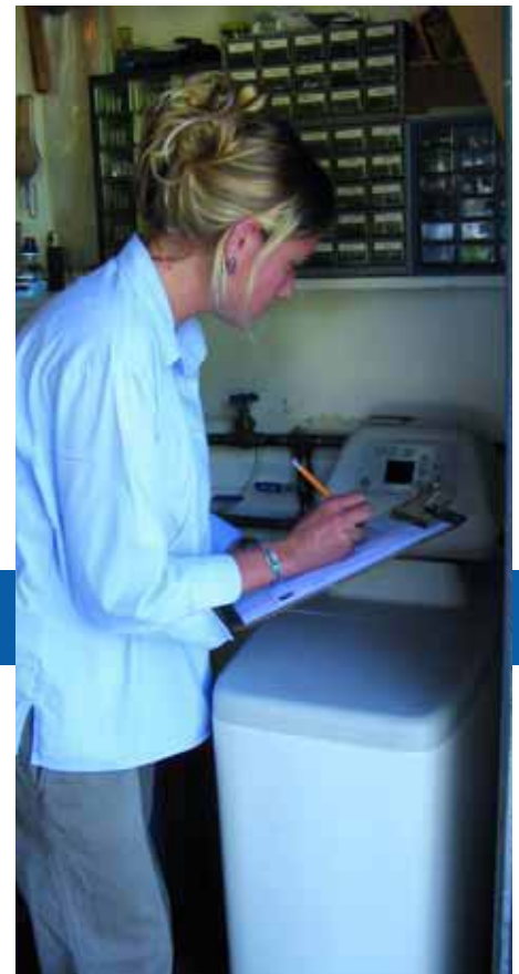
Right: A demand-initiated, regenerational water softener, for which county residents received rebates of $150. Based on monthly water consumption data, the annual water savings from this successful pilot project is estimated to be more than 1.3 million gallons.
