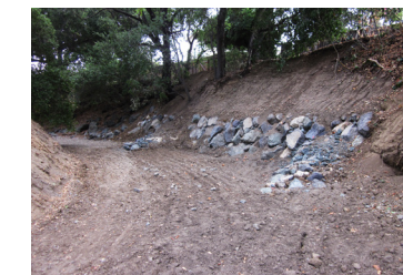
After Erosion Repair
