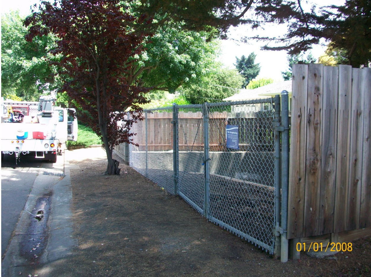
2" Galvanized fence fabric with "No Trespassing" sign installed on gate
