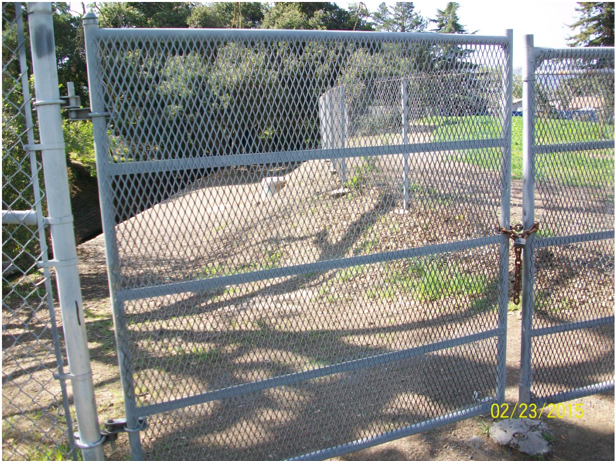
\frac{3}{4} " #9 flat expanded metal attached to gate frames
