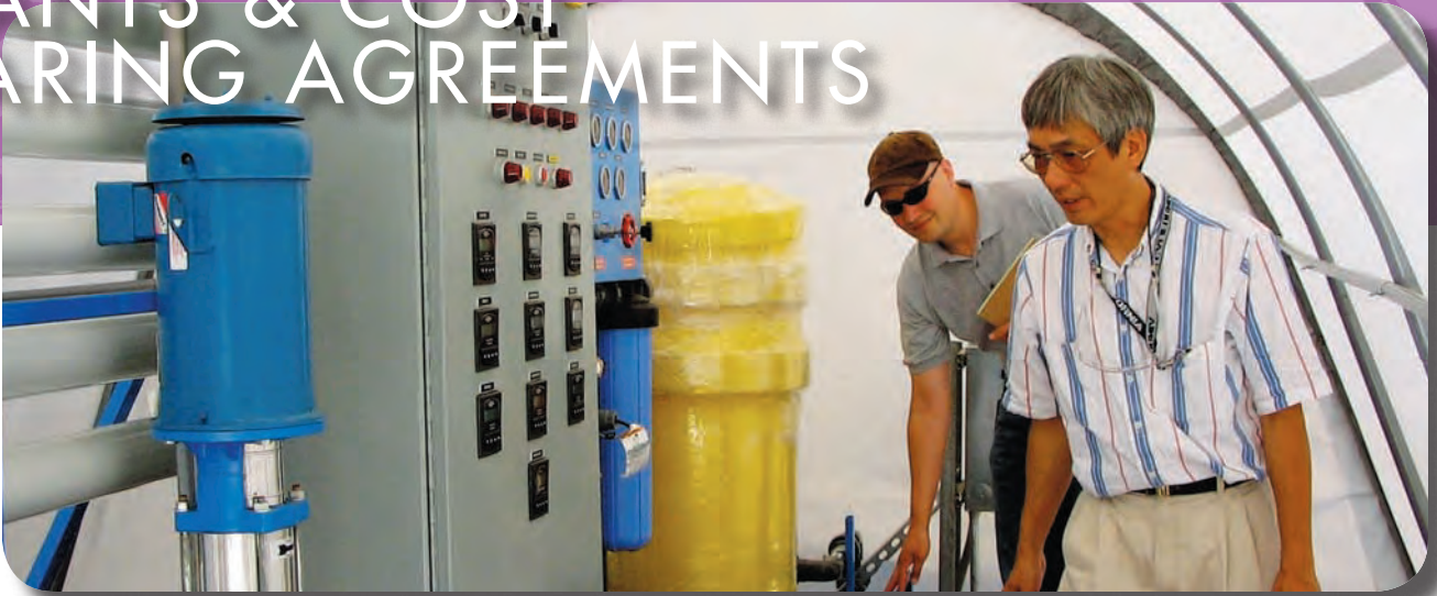
Ray Wong examines reverse osmosis treatment pilot plant.
