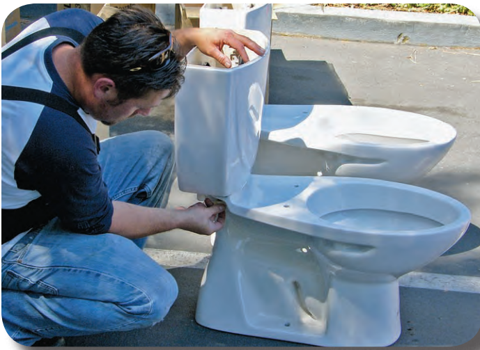
A technician assembles an HET for an apartment complex
