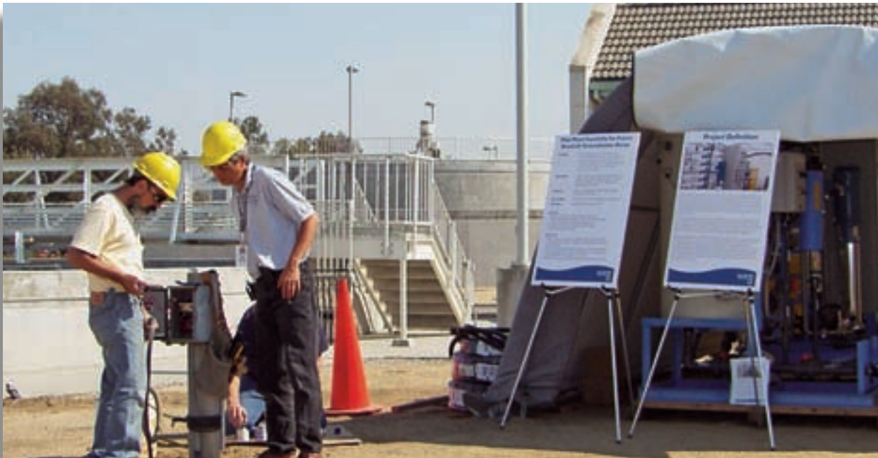
Pilot brackish groundwater desalination effort in Gilroy using reverse osmosis membrane technology.
