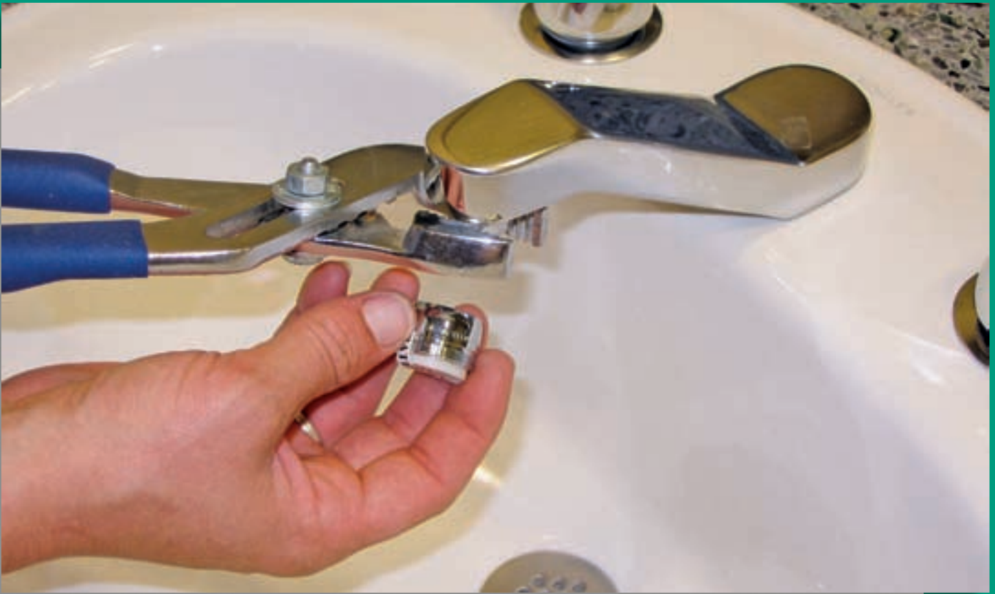
Replacing an old faucet aerator for an efficient one.
