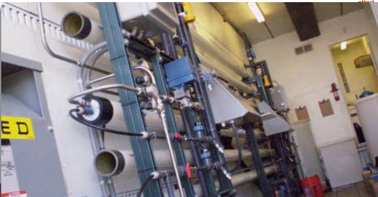
Pilot Desalination at Mallard Slough, East Contra Costa. Part of district's Regional Desalination Project (RDP) effort
