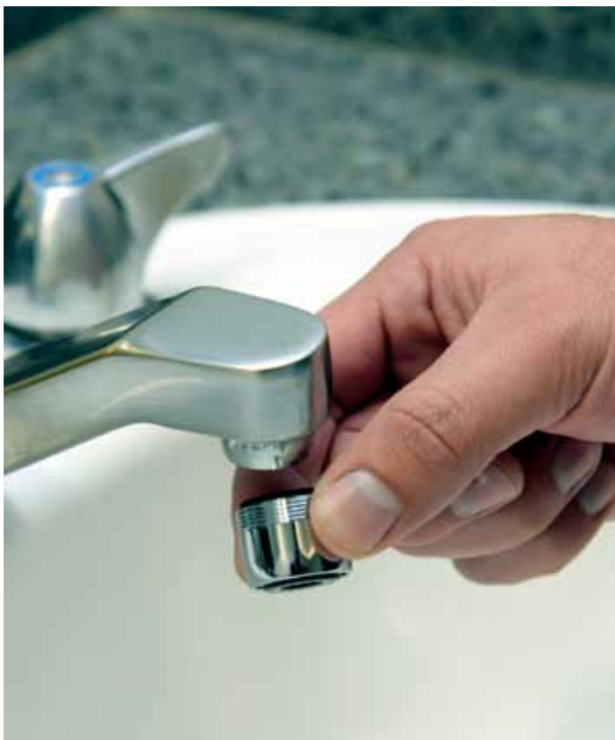
Installing a low-flow faucet aerator on a commercial bathroom faucet.
