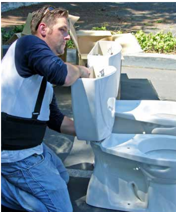
A technician installs a high-efficiency toilet at an apartment complex.
