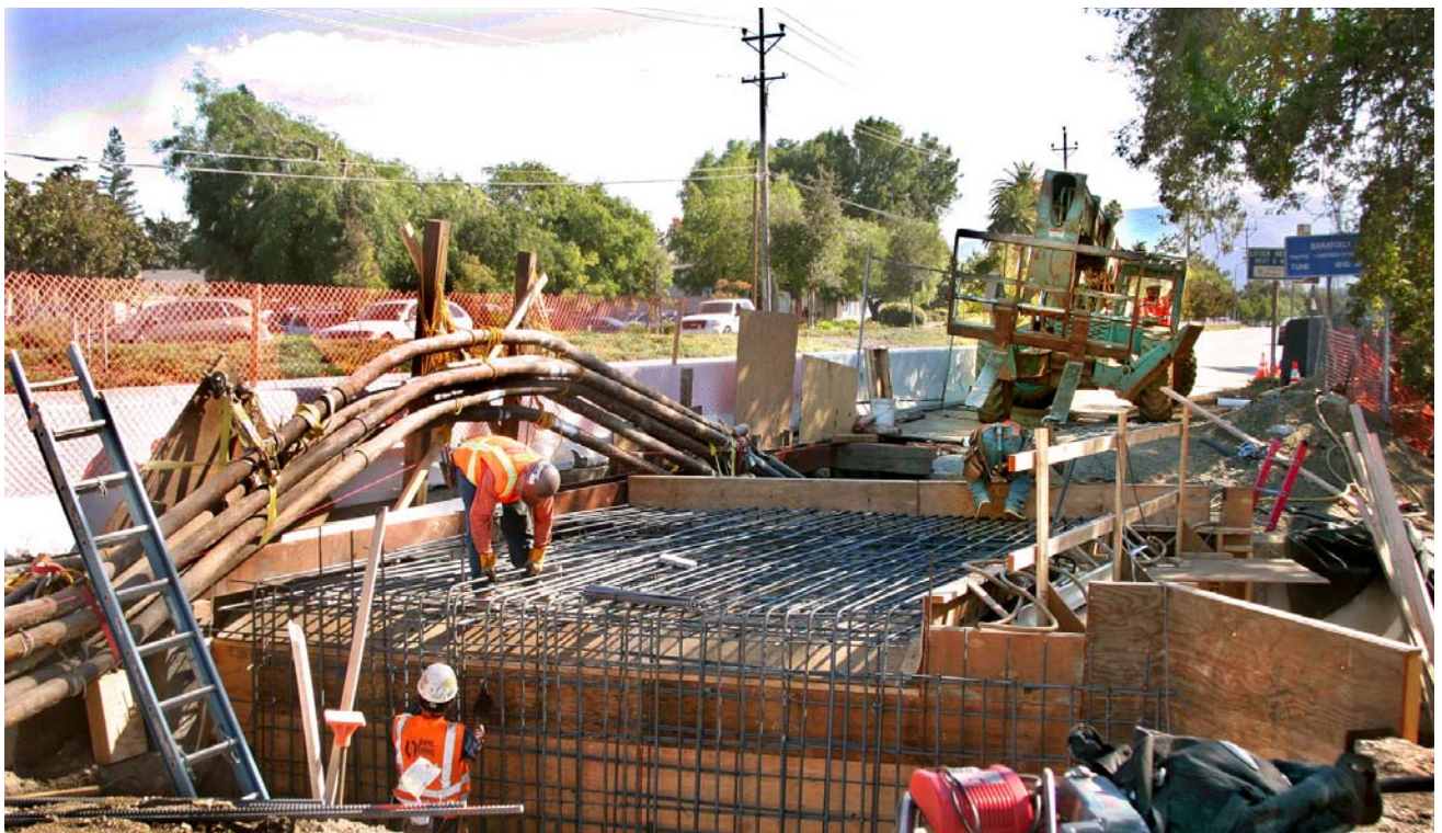
Calabazas Creek project work in full swing
