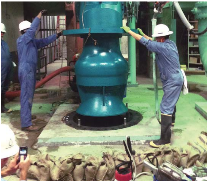
Maintenance work at the Rinconada Water Treatment Plant
