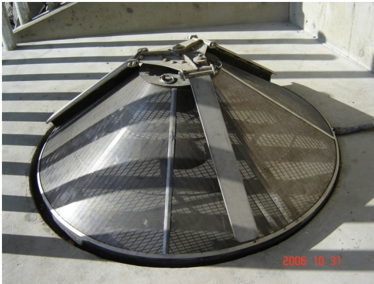
Figure 4. Typical Cone-Shape Fish Screen
