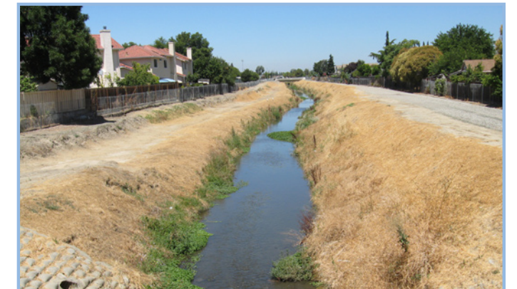
Lower Silver Creek (Reach 6, near Cunningham Ave) creek banks will be stabilized and flood conveyance will be improved.
