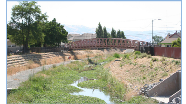
Lower Silver Creek (Reach 3) completed in 2006; enhanced habitat and vegetation, and improved maintenance.
