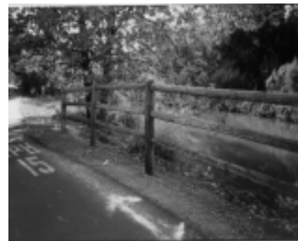
FIGURE: Typical three-rail fence as used along Los Gatos Creek at Lark Avenue
