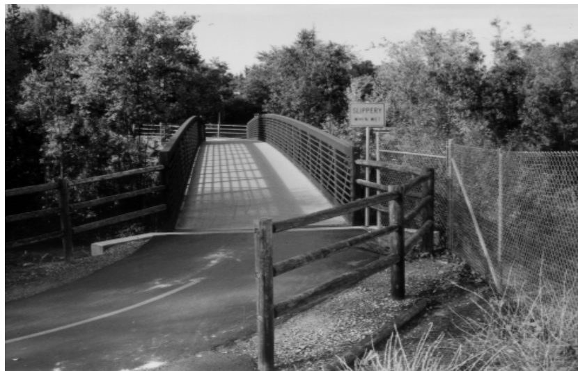
FIGURE: The chain link fence located at this Los Gatos Creek bridge landing would be less visible but still effective if it was placed a few feet downhill and away from the more decorative three rail fence.
