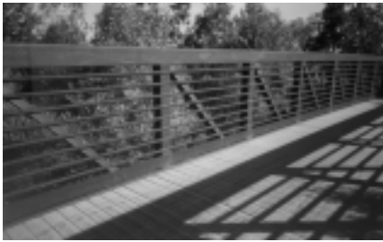
FIGURE: Recycled plastic lumber bridge decking at Los Gatos Creek
