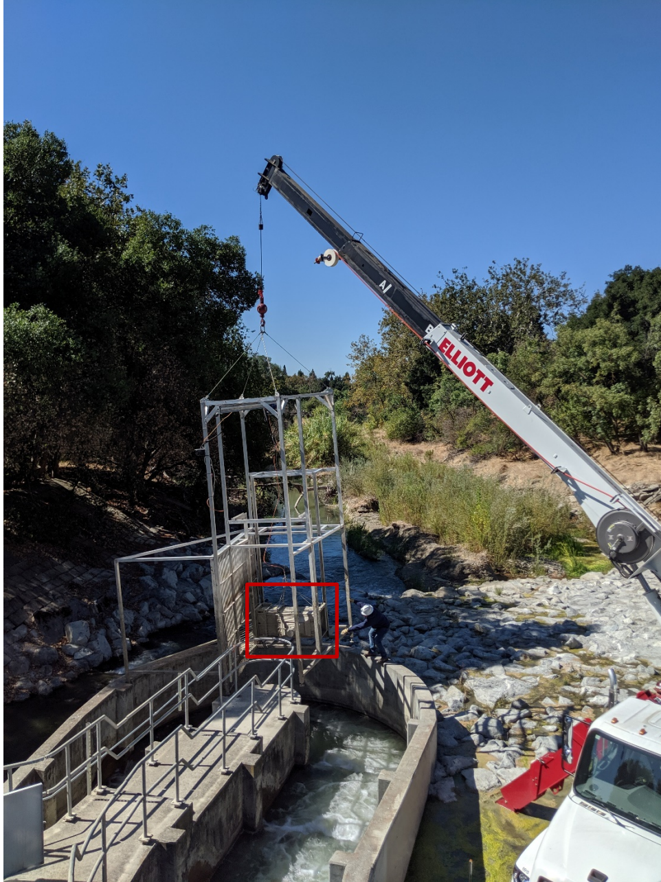
Figure 2. Installation of the Vaki Riverwatcher system in the Coyote Creek Fishway on October 2, 2019. The red box indicates the fish counter.
