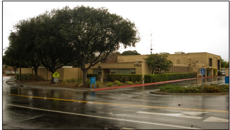
Existing Maintenance Building
