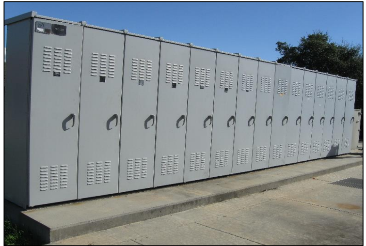
Motor control center switchboard
