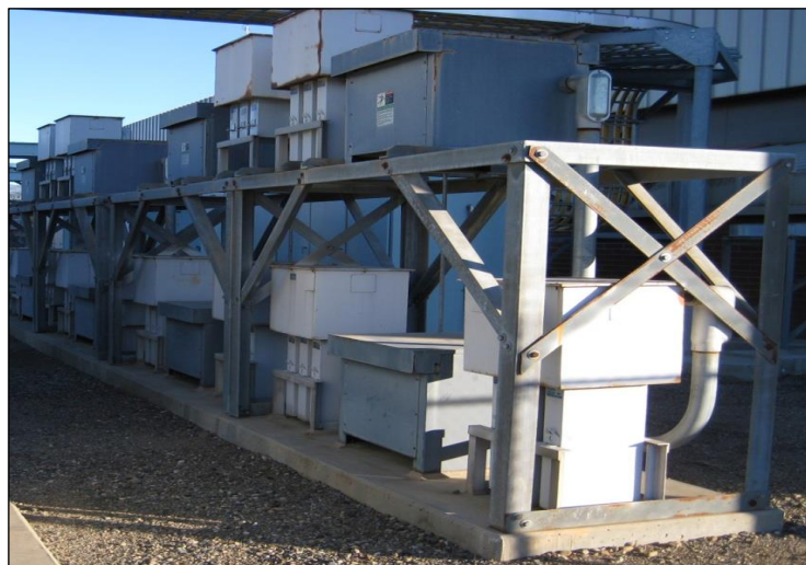
ASD motors at the Coyote Pumping Plant
