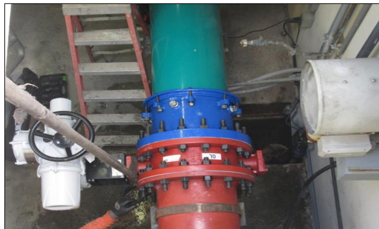
A typical rehabilitated line valve assembly
