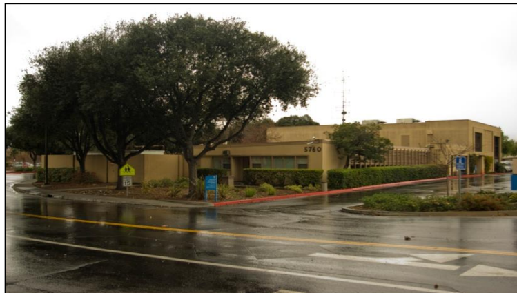
Existing Maintenance Building
