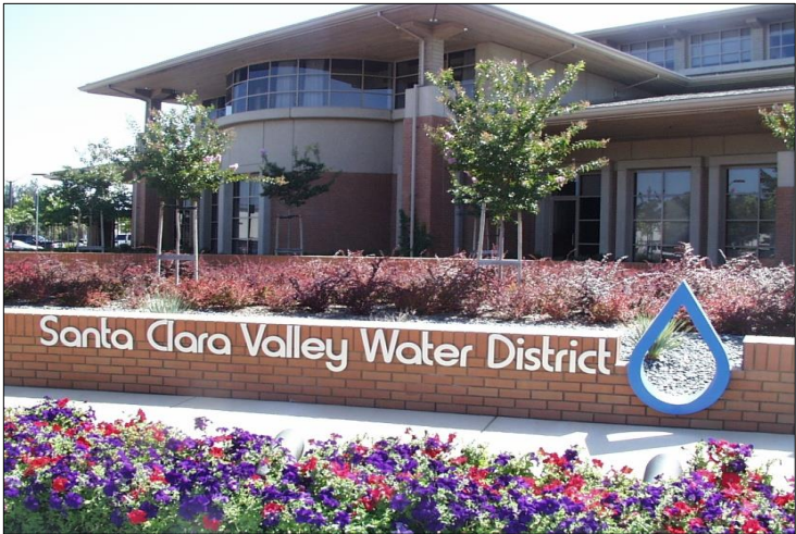
Front view of the Headquarters building at the Almaden Campus
