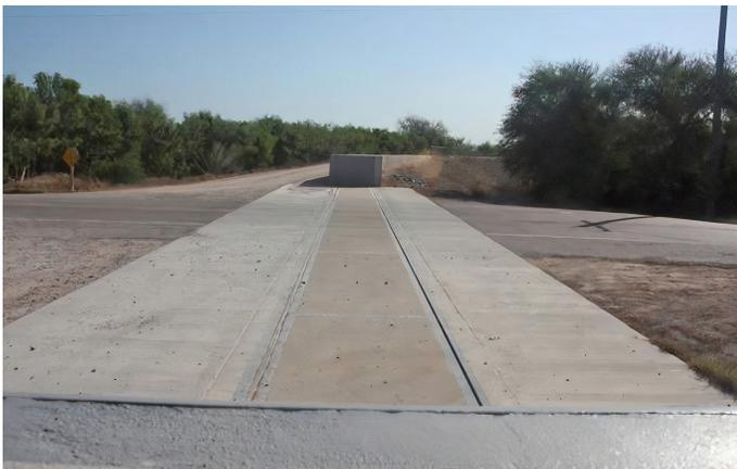
Image of an actual barrier installed in the embedded condition.
