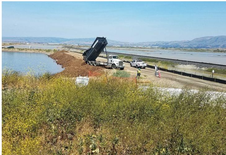
Soil was delivered to Pond A12 for use on future levee construction.
