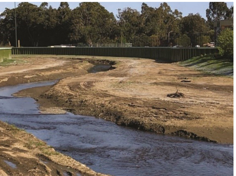
San Francisquito Creek floodwall, February 2019.
